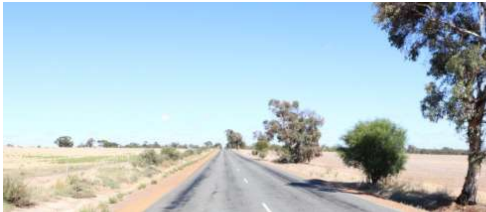
Figure 2.12 Site A2, Wickepen-Pingelly Road
