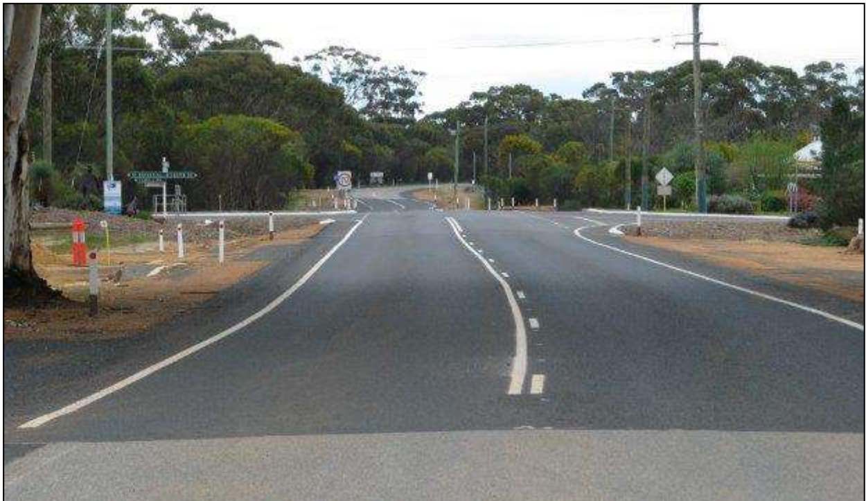
Figure 10: Example of lane marking stereotypes listed as 3 and 4 for asphalt; (3) broken-barrier centrelines (out of page) and (4) barrier-broken centrelines (into page).
