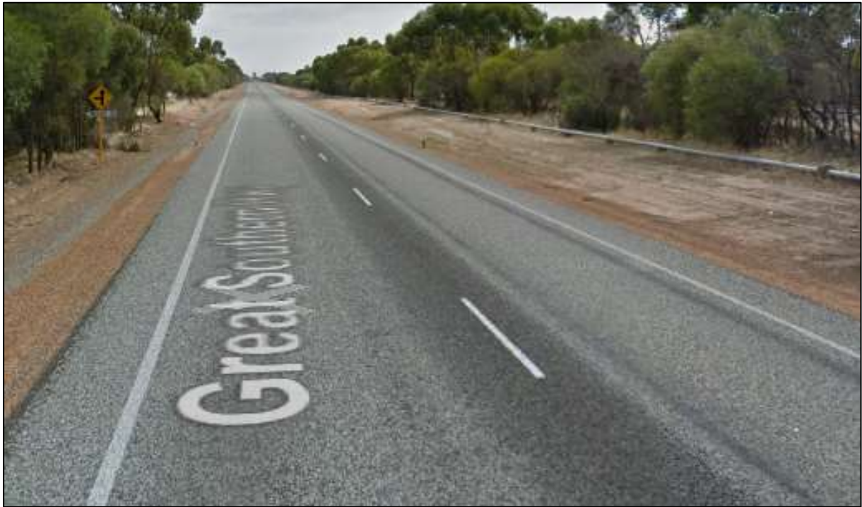
Figure 5 : Example of line marking stereotypes listed as 1 and 4 for sealed pavement; (1) solid edge lines with sealed shoulders and (4) a broken centreline.
