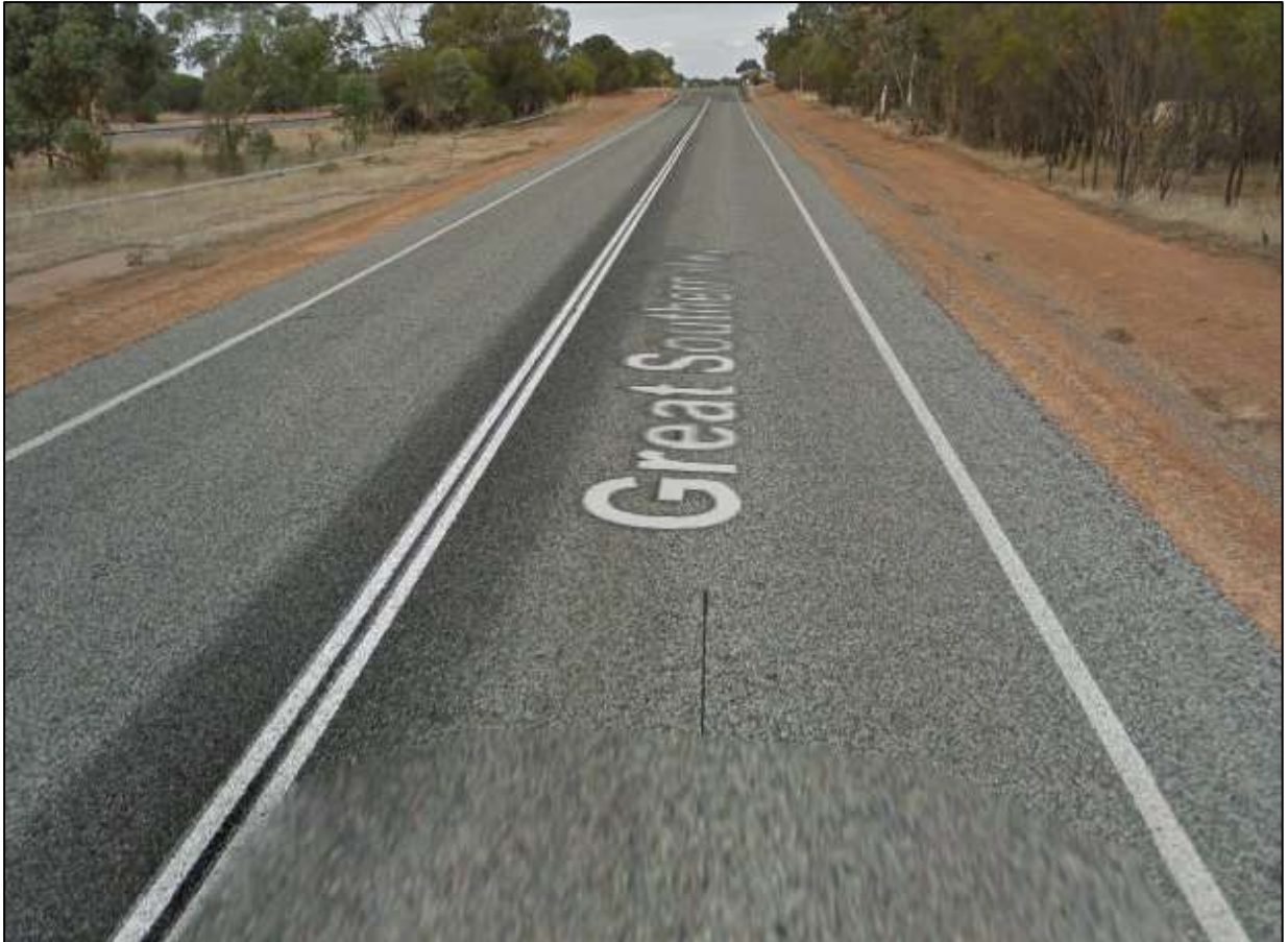
Figure 7: Example of line marking stereotype listed as 3 for seal pavement; double barrier centrelines.
