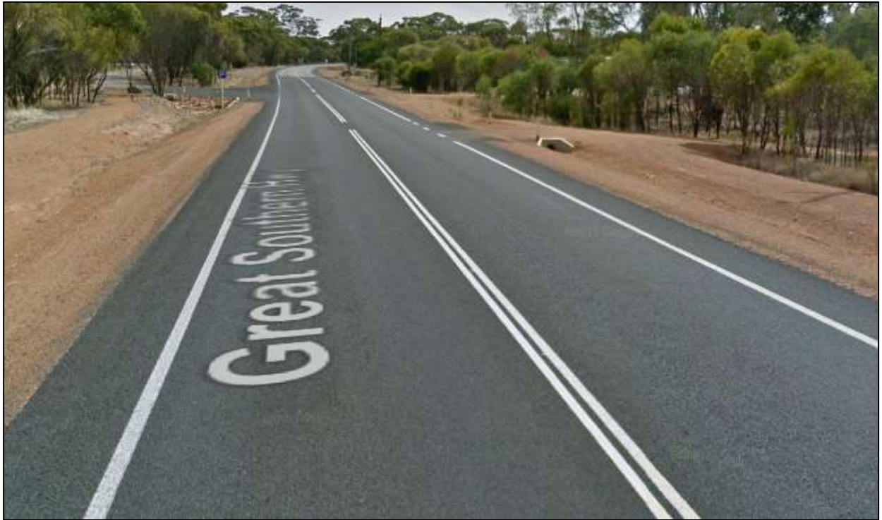
Figure 9: Example of line marking stereotypes listed as 1 and 2 for asphalt; (1) solid edge lines with wide shoulders, and (2) a double barrier centreline.
