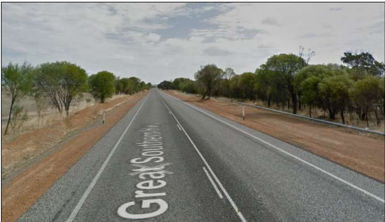
Figure 8: Example of line marking stereotypes listed as 5 and 6 for sealed pavement; (5) broken-barrier centrelines (into page) and (6) barrier broken centrelines (out of page).
