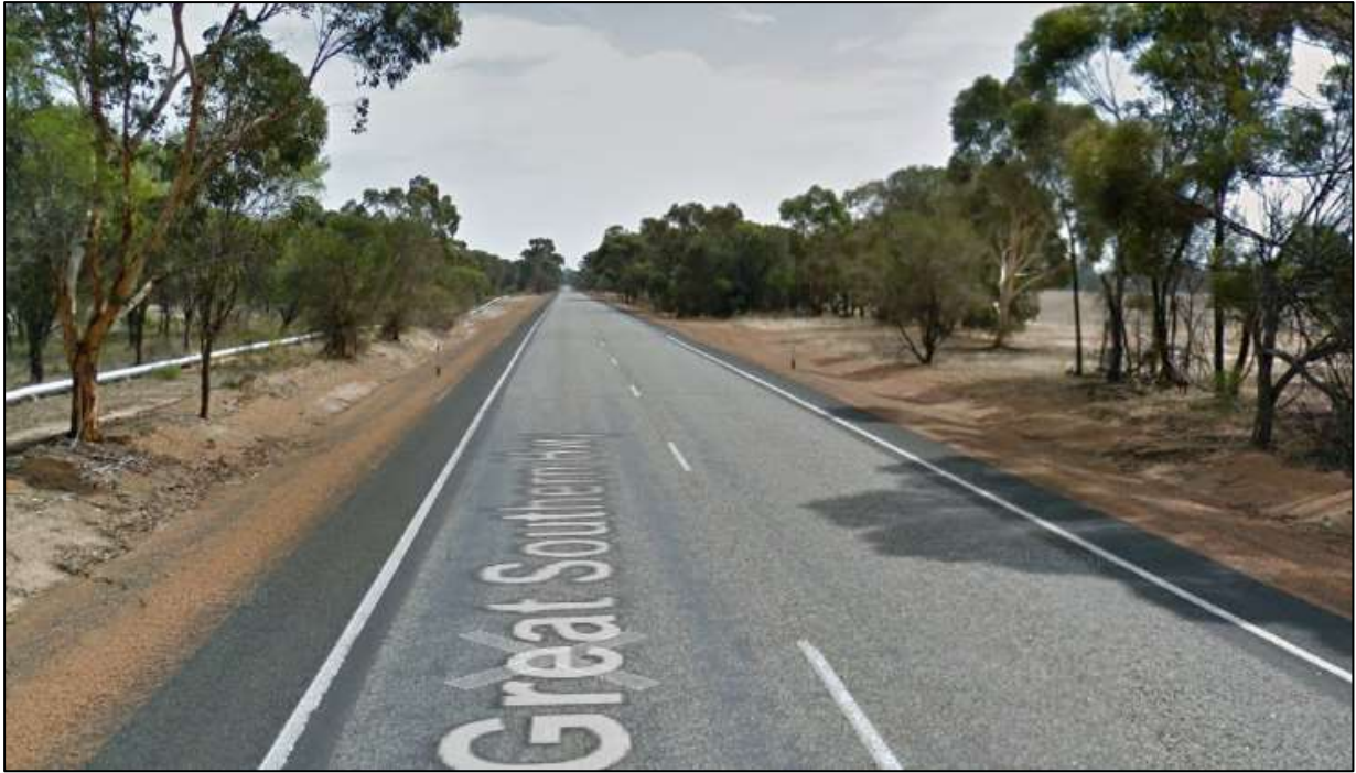
Figure 6: Example of line marking stereotype listed as 2 for sealed pavement; solid edge lines with sealed, dark shoulders that encroach into the carriageway.
